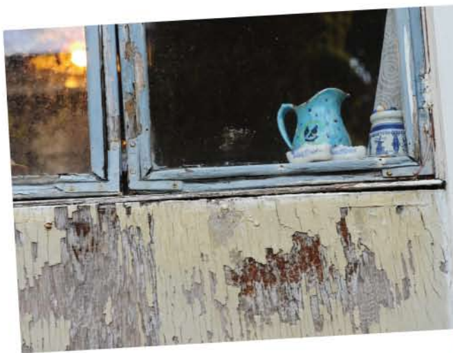
Wally Jensen 809 Lawrence Road, kitchen window San Mateo, California
